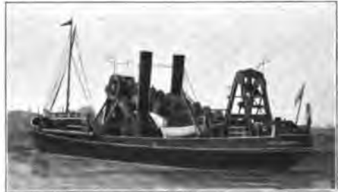
Fig. 8.—Twin-screw hopper-dredger, "Percy Sanderson," built for the European Danube Commission by Wm. Simons & Co.
