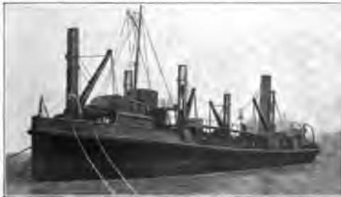
Fig. 9.—Twin-screw grab-dredger, "Miles K. Burton," built for the Mersey Docks and Harbour Board by Wm. Simons & Co.
