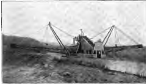
Fig. 5.—Dredger constructed for the Lake Copais Co. by Hunter & English.
